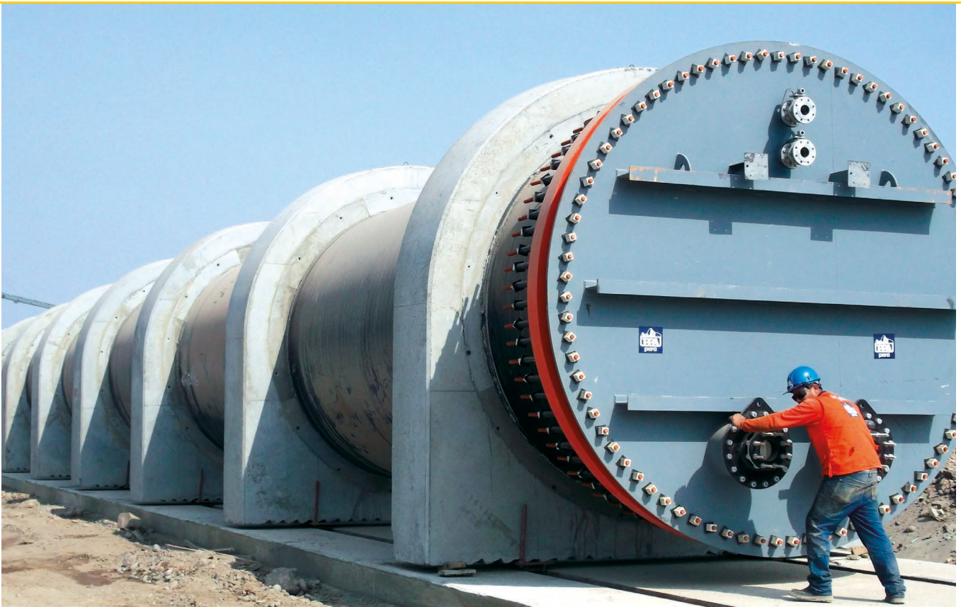
Preparing an outfall pipeline string DN/ID 3000 mm
