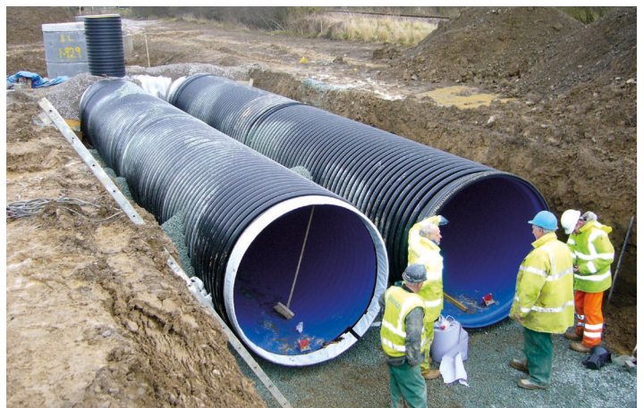
Installation of stormwater system DN/ID 1800 mm
