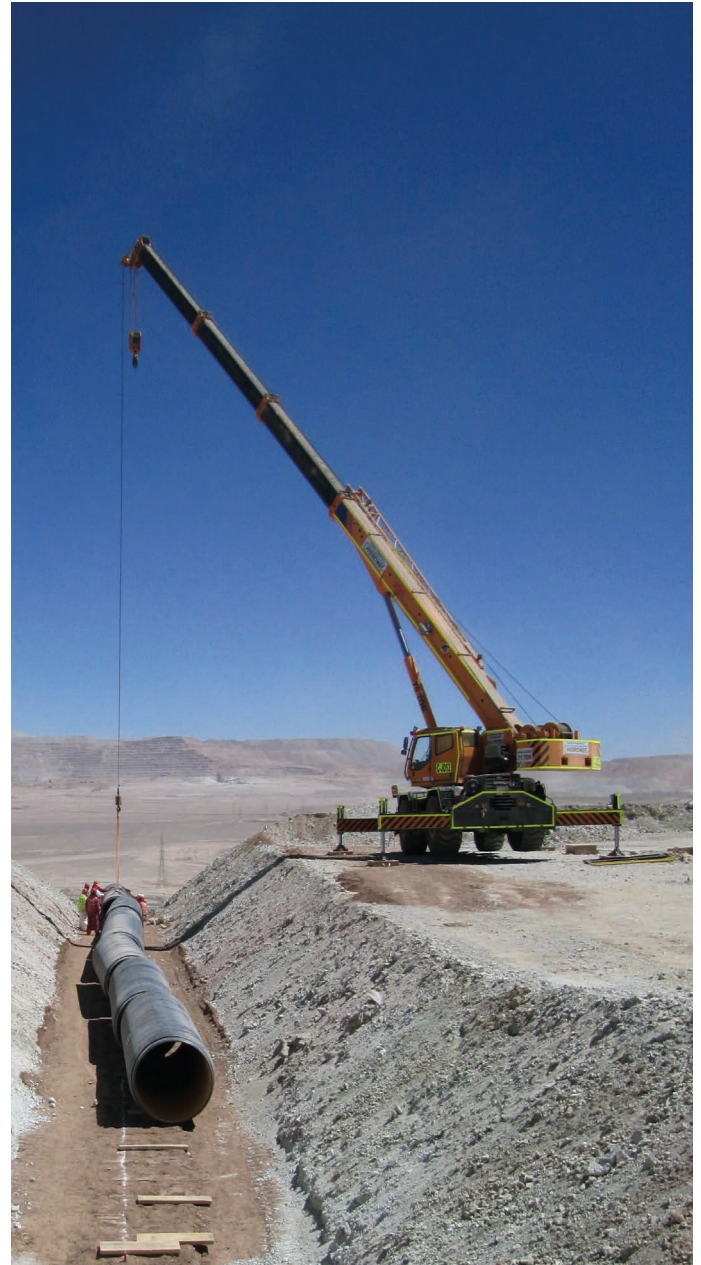
Installation of pipes DN/ID 1800 mm in a mining project for slurry
