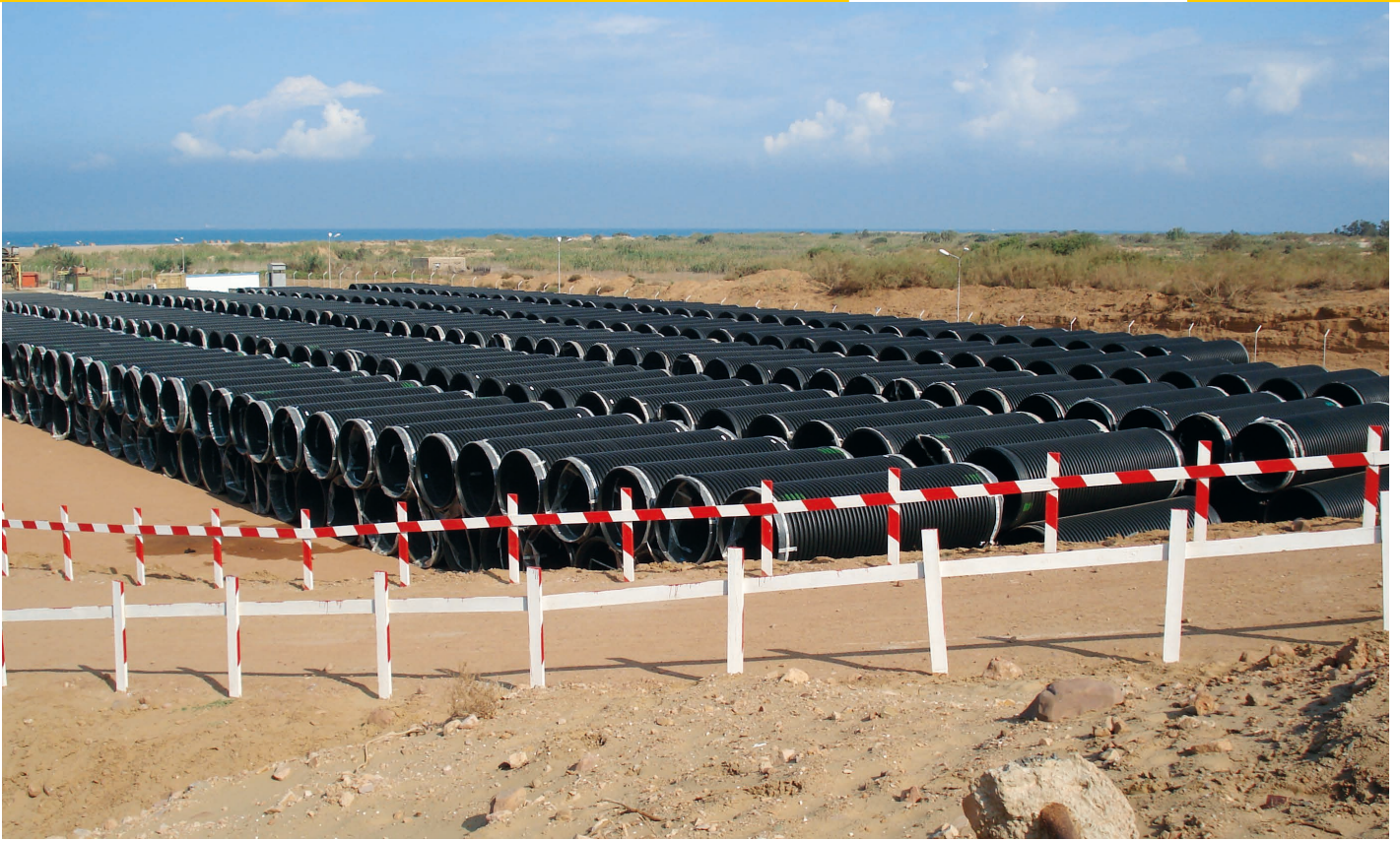
Open storage of pipes DN/ID 1600 mm
