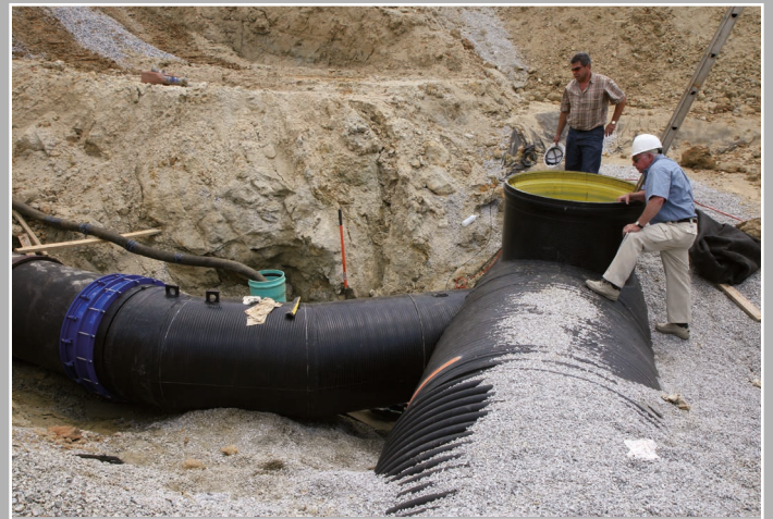
Installation of pipes DN/ID 2000 mm, with manhole & bench
