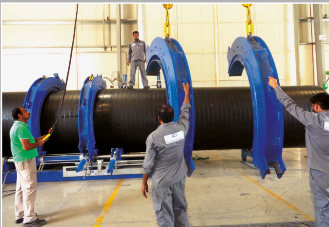
Butt-welding of pipes DN/ID 1800 mm
