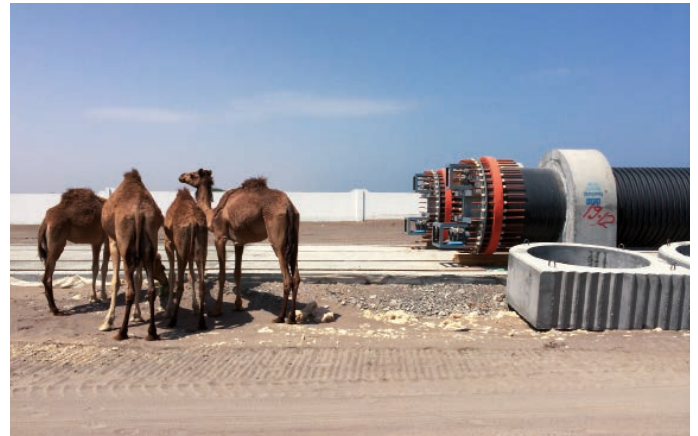
Pipe of DN/ID 2000 mm installation in a hot environment
