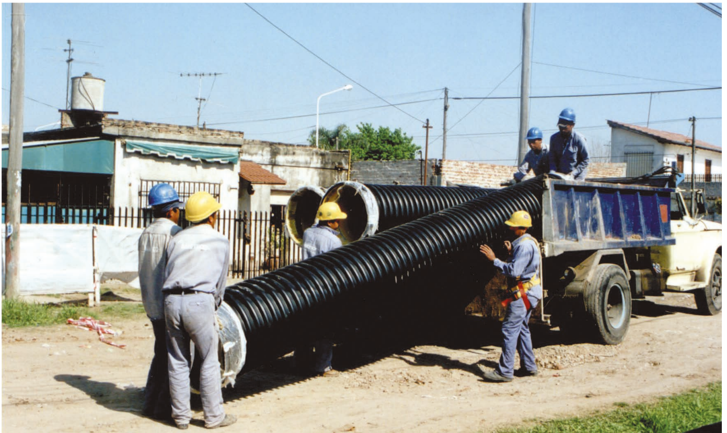
Light weight pipe - Manual unloading of a pipe DN/ID 600 mm
