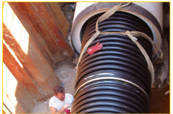
DN/ID 1200 mm relining of a concrete pipe
