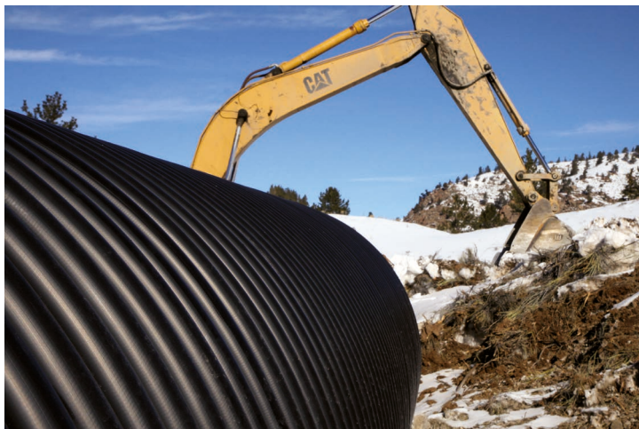
Installation of pipe with DN/ID 1600 mm during low temperature
