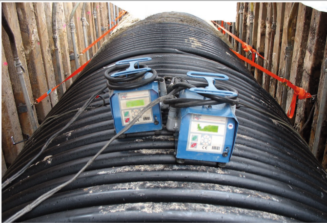
Electro-Fusion joint DN/ID 1800 mm
