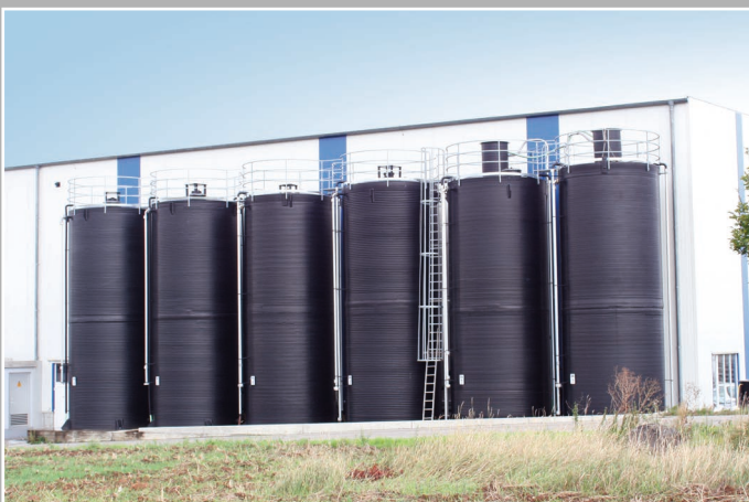
Industrial storage system „silos“
