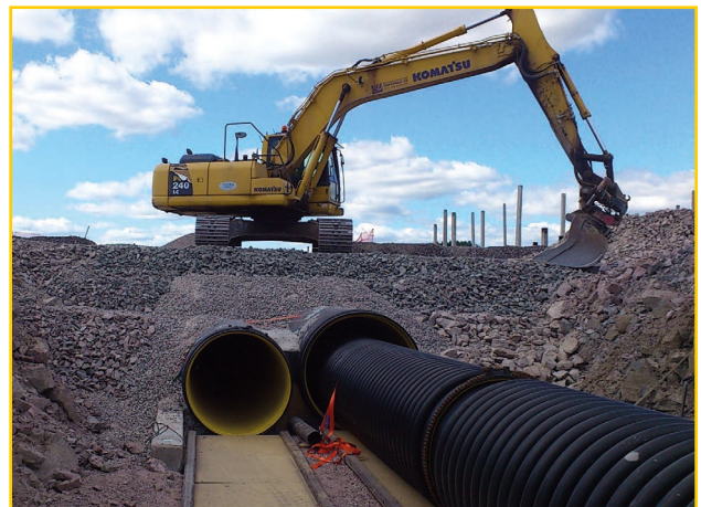
Installation of two pipe strings DN/ID 1200mm+ DN/ID 1400 mm
