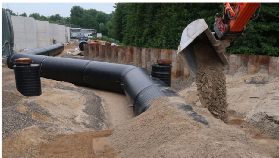
Fig. 12 - Installation of sand in the pipeline zone
