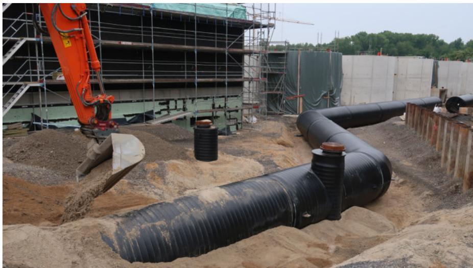
Fig. 10 - Installation of sand in the pipeline zone
