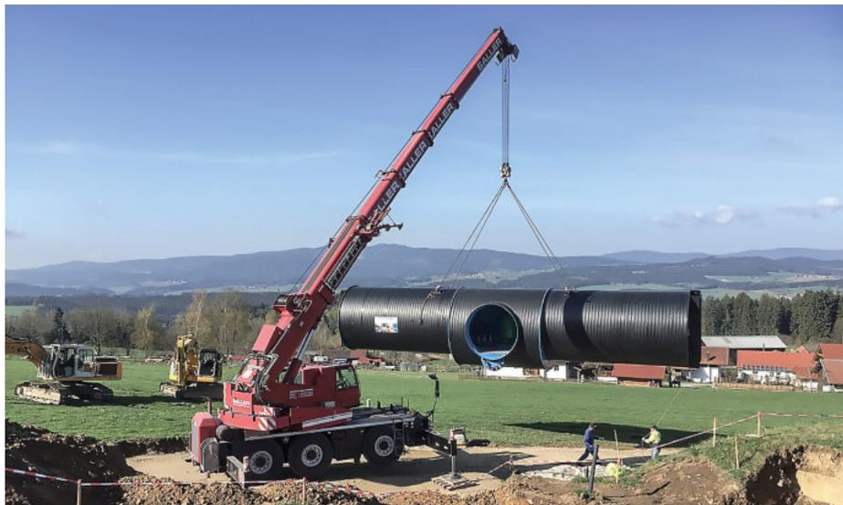
Fig. 4 - PE system container -  $2 \times 40 \text{ m}^3$  - delivery in one piece
