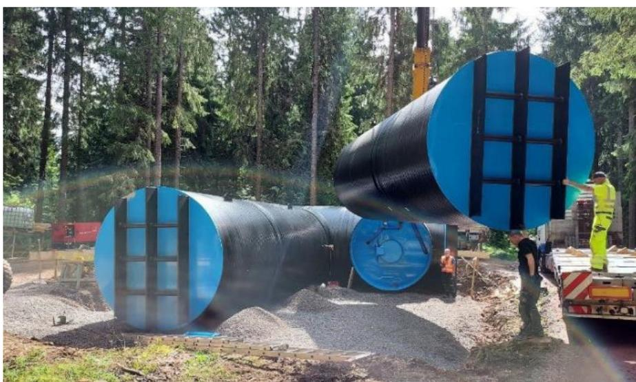
Fig. 5 - Prefabricated container made of PE -  $2 \times 60 \text{ m}^3$  - Delivery in 3 individual parts
