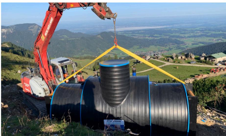
Fig. 7- Installation of the „Steinlinalm“ tank - 2 x 3 m<sup>3</sup> with central valve chamber
