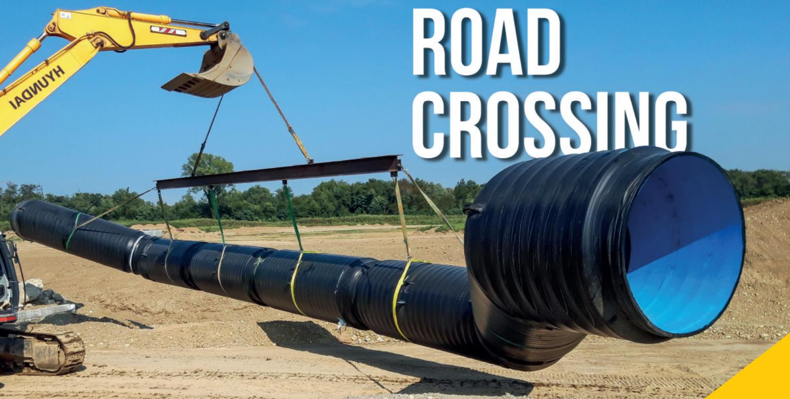
A large black plastic pipe is being lifted by a yellow excavator at a construction site. The pipe is supported by a metal beam and yellow straps. The excavator's arm is visible on the left, and the pipe extends across the middle of the frame. The background shows a clear blue sky and some greenery.
